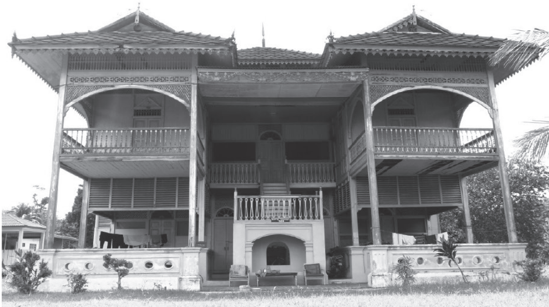
Figure 7: Baitul Rahmah, Kuala Kangsar: A hybrid masonry plinth and column base fused with timber columns, portico, side balconies, and decorative eaves
